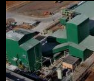
Ammonium Nitrate Facility
