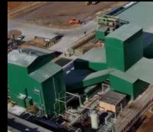
Ammonium Nitrate Facility
